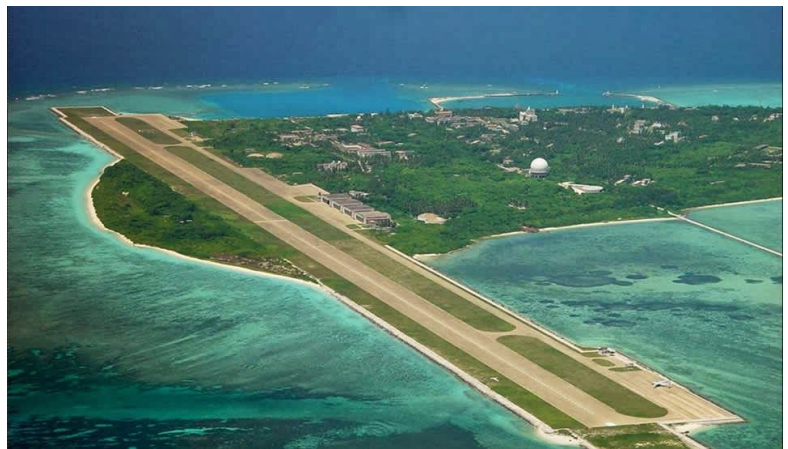
Aerial view of Woody Island
